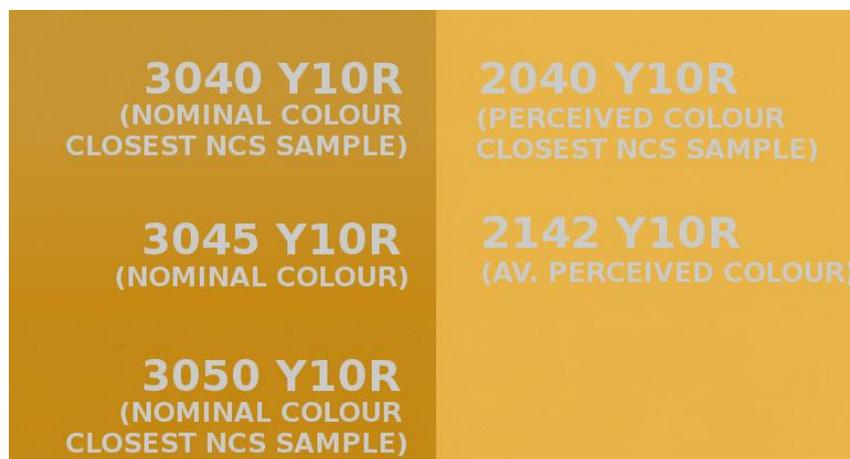
Figure 26: The nominal colour (left) and the averaged perceived colour (right) of façade E (Table 4).
